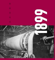
The American rotary kiln, invented by Aalborg Portland's Poul Larsen, built for the first time in Europe, as two new rotary kilns are installed at the Rørdal factory. The production capacity is significantly upgraded.
