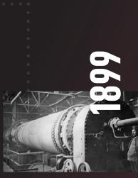
The American rotary kiln, invented by Aalborg Portland's Poul Larsen, built for the first time in Europe, as two new rotary kilns are installed at the Rørdal factory. The production capacity is significantly upgraded.
