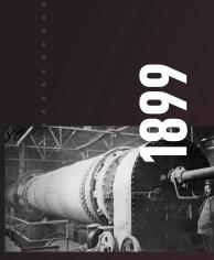
The American rotary kiln, invented by Aalborg Portland's Poul Larsen, built for the first time in Europe, as two new rotary kilns are installed at the Rørdal factory. The production capacity is significantly upgraded.
